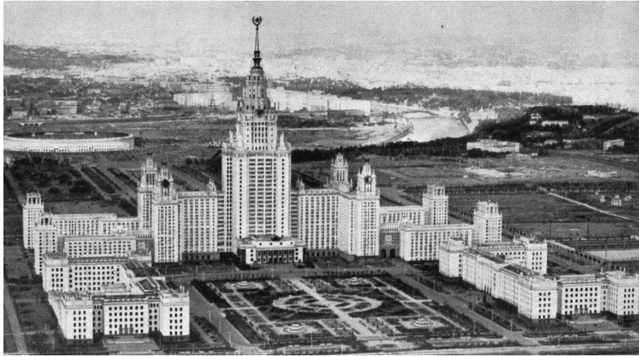
Lev Rudnev, Moscow State University, Moscow, 1949–1953. From Oltarzhevsky, The Construction of High-Rise Buildings in Moscow , 28.
