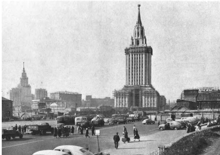
Leonid Polyakov, Hotel Leningrad, Moscow, 1949–1954. From Oltarzhevsky, The Construction of High-Rise Buildings in Moscow , 140.
