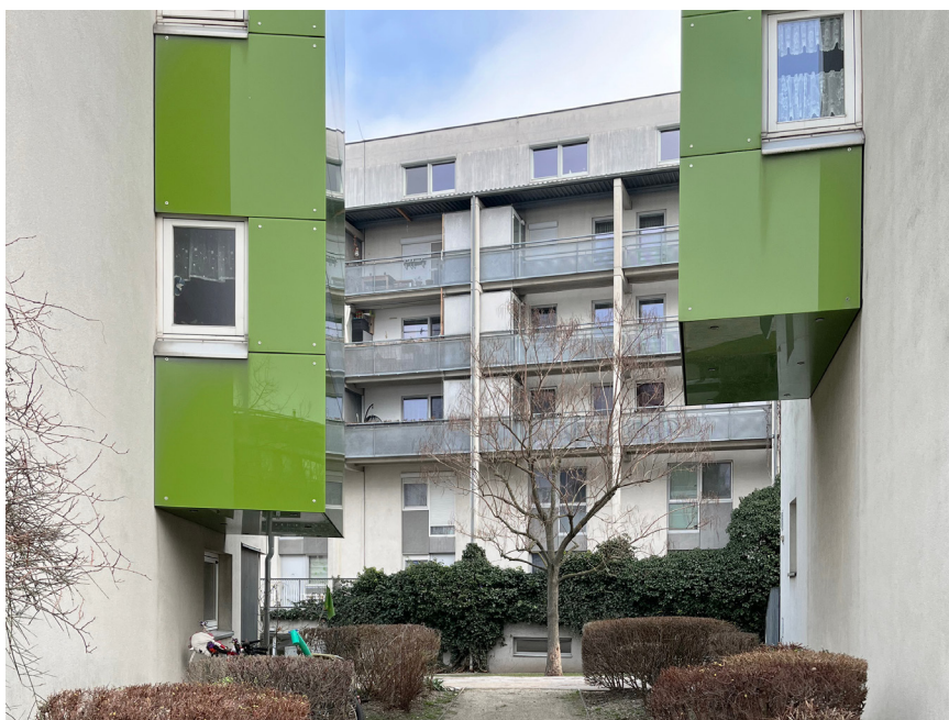
Site view of Frauen-Werk-Stadt, unit B in the foreground and unit A in the background. Photo by the author, 2023.
