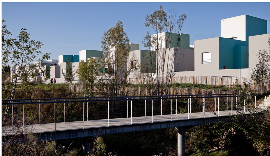
50 social housing units, Nantes, 2007. Photograph by Pierre-Yves Brunaud.
