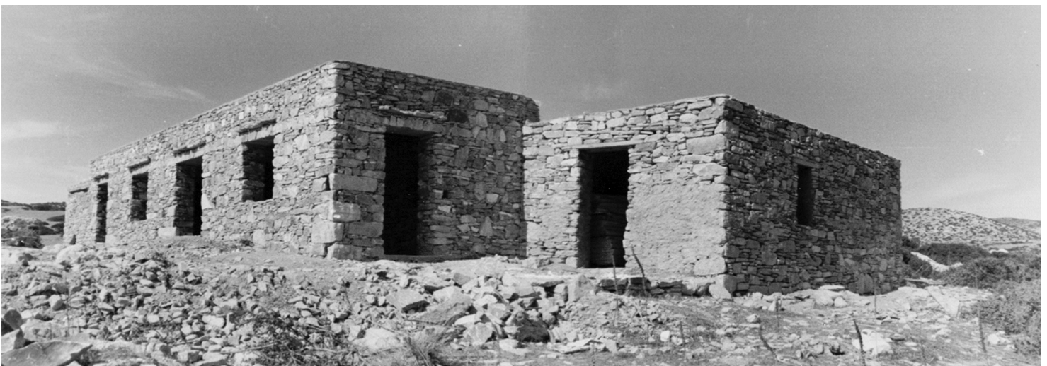
Villa T, under construction, Antiparos, 1982. Courtesy Katerina Tsigarida Archive.
