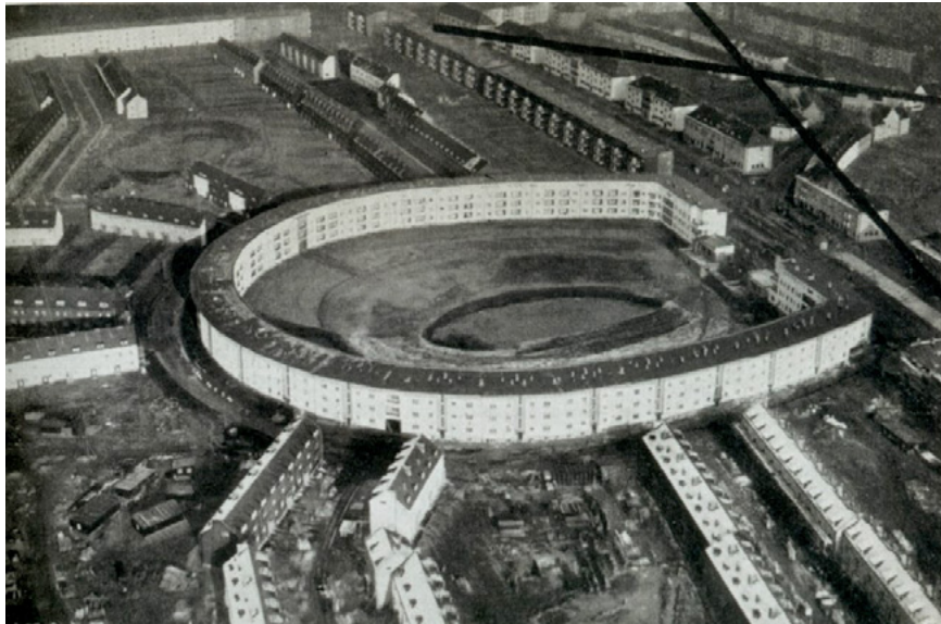
Aerial view of the Hufeisensiedlung in Berlin, designed by Bruno Taut and Martin Wagner, built between 1925 and 1931.
