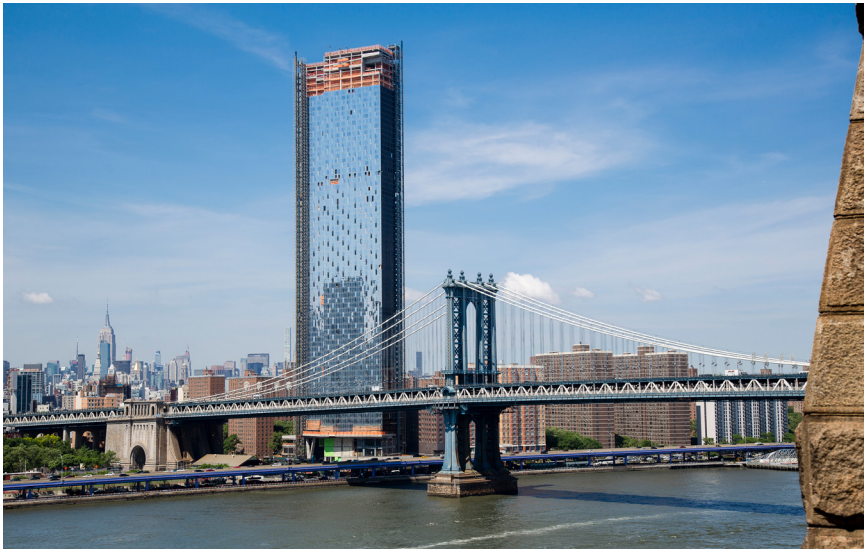
Partial view of One Manhattan Square over Manhattan Bridge.
