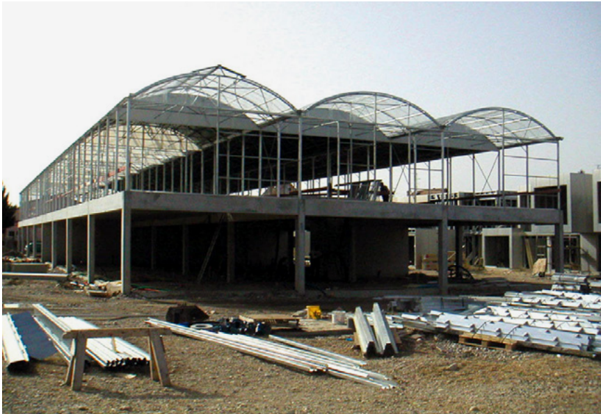
Collective housing during construction. Cité Manifeste, Mulhouse, 2005. © Lacaton & Vassal Architectes.
